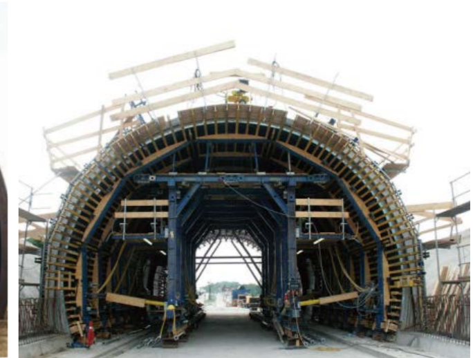
Timber Formwork Tunnel Trolley 木模体系隧道台车
