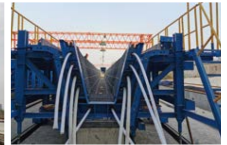
Prefabricated Box Girder (Hydraulic) 预制箱梁(液压)
