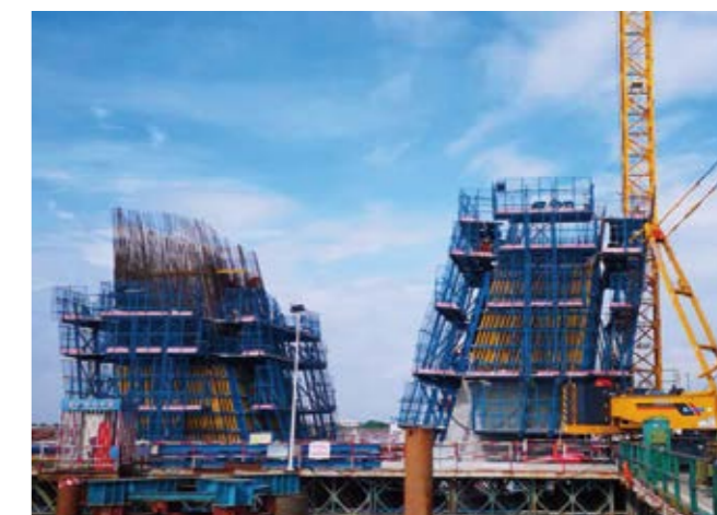
Climbing Formwork for Pier 墩柱爬模
