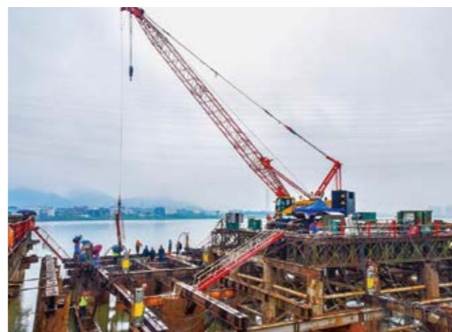
Steel Box Cofferdam with Bottom 有底钢套箱
